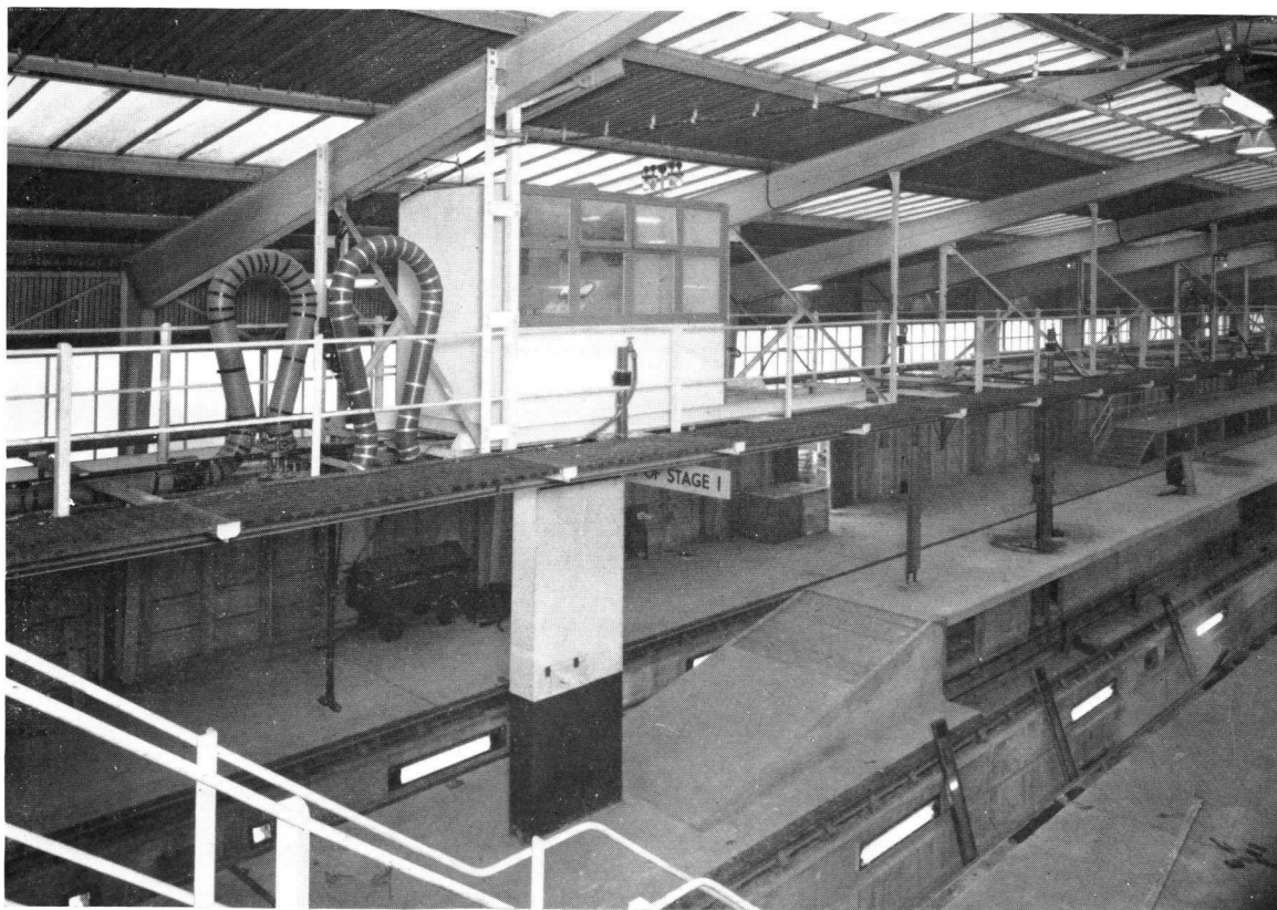
ONE OF THE CONTROL CABINS
