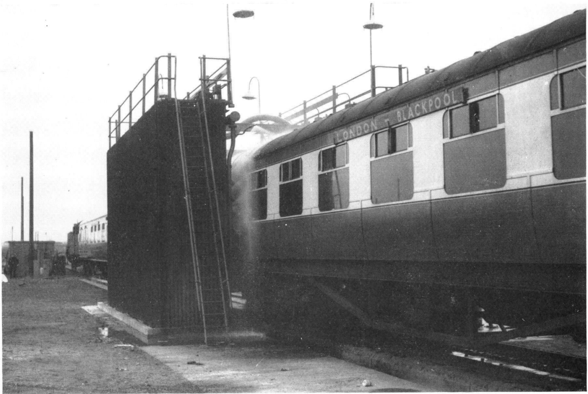
CARRIAGE WASHING PLANT IN ACTION
